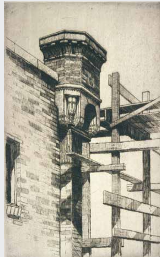
Gordon Gilkey (American, 1912–2000). University of Oregon Library Construction , 1936. Etching, 10 3/8 x 6 3/4 in. Allocated by the U.S. Government Commissioned through the New Deal art projects
